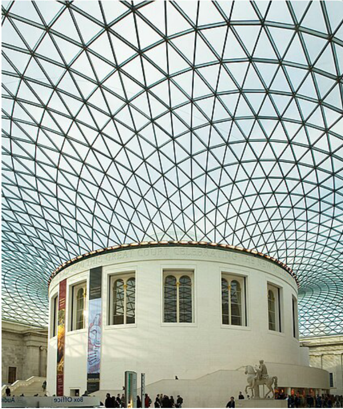
Figure 1 Lattices spanning the roof of the Great Court of the British Museum, London.
